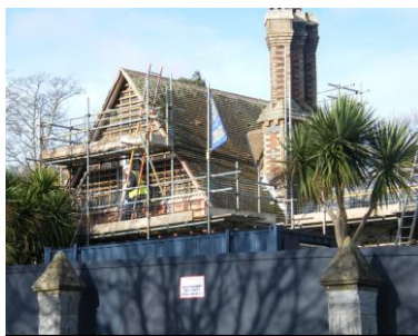
Devonport Park Lodge, prior to work starting.
